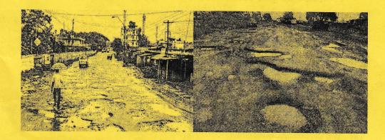
causes fatal accidents –extensive damage to vehicles-traffic jams-absence of proper drainage systems-low quality material used-should be priority for any Government
